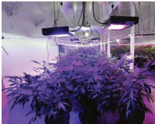
This garden uses LED supplements with HPS to create broader spectrum.
